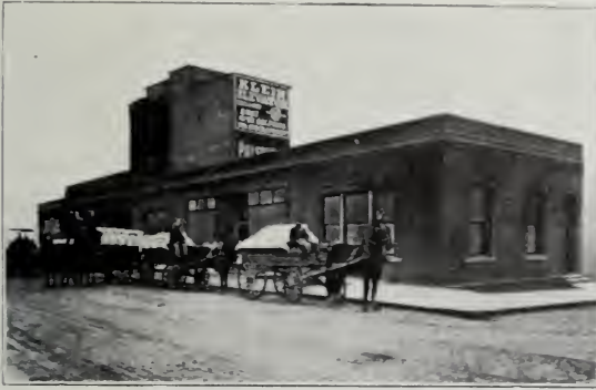
The Klein Elevator as rebuilt after the fire.
