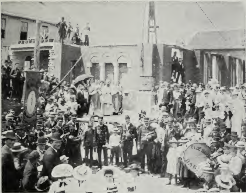
St. Benedict's Church in construction, 1895.
