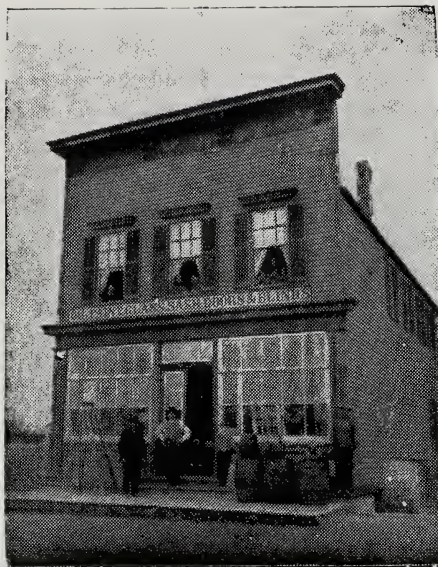
Northwest Corner of York and Western This building was erected in 1855 by Herman Schmitt. In later years it was much improved and occupied by the Schmitt Brothers Department Store.
