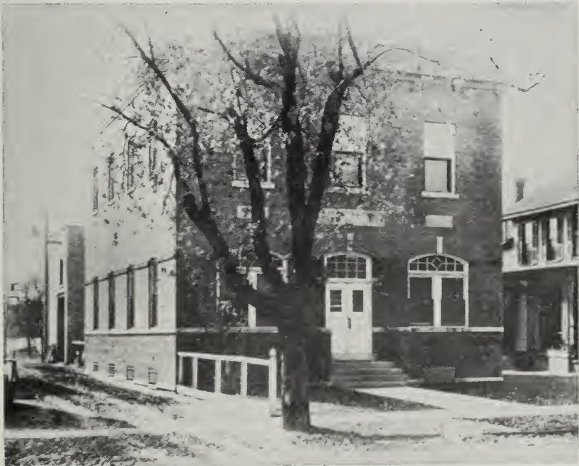
Home of the Chicago Telephone Company, 1905 After remodeling this building became the Elks Club.
